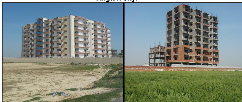
Figure 04: A recently constructed apartment building (left) and an institutional building (right) under construction after conversion of prime agricultural lands in the fringe of Aligarh city.
